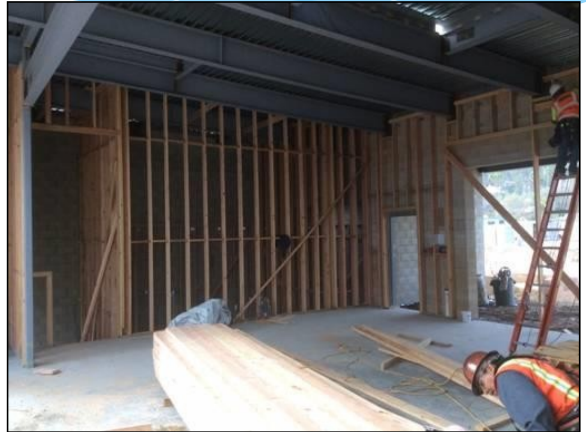
Interior Wall Framing at Stage
