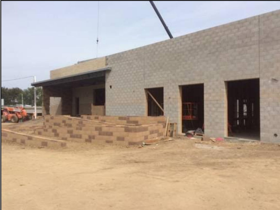
MP Bldg: West Elevation (from South)
