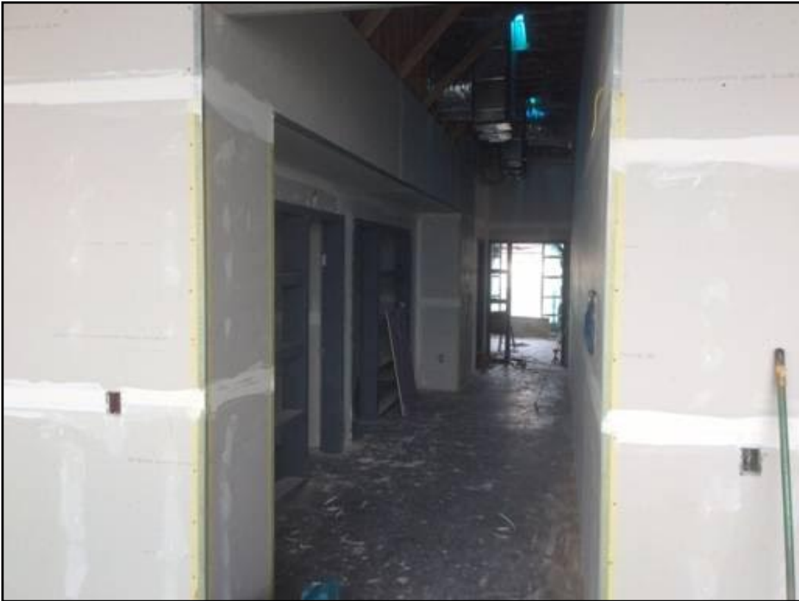
Admin Bldg: West Hallway
