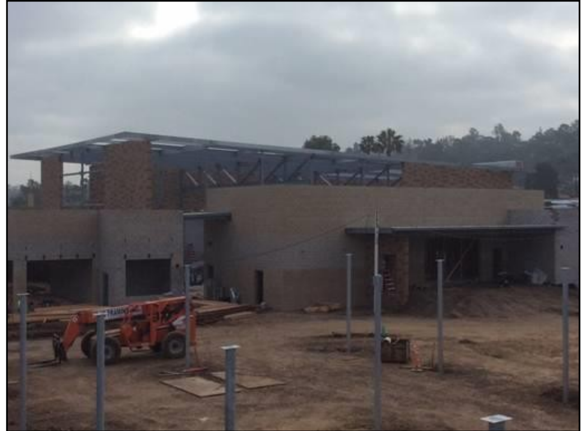
MP Bldg: NW Elevation
