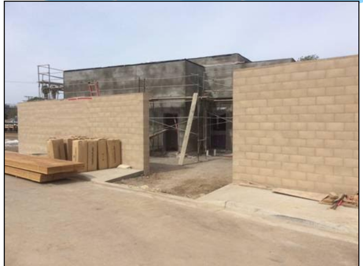
Food Services Bldg: South Elevation
