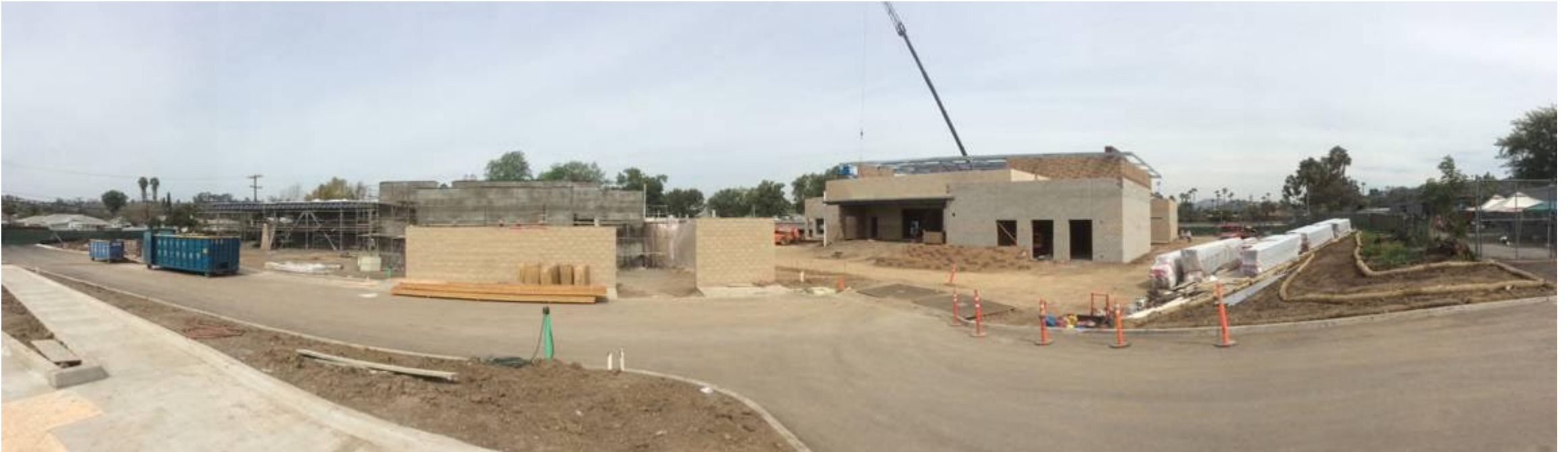
Overall Construction Site
