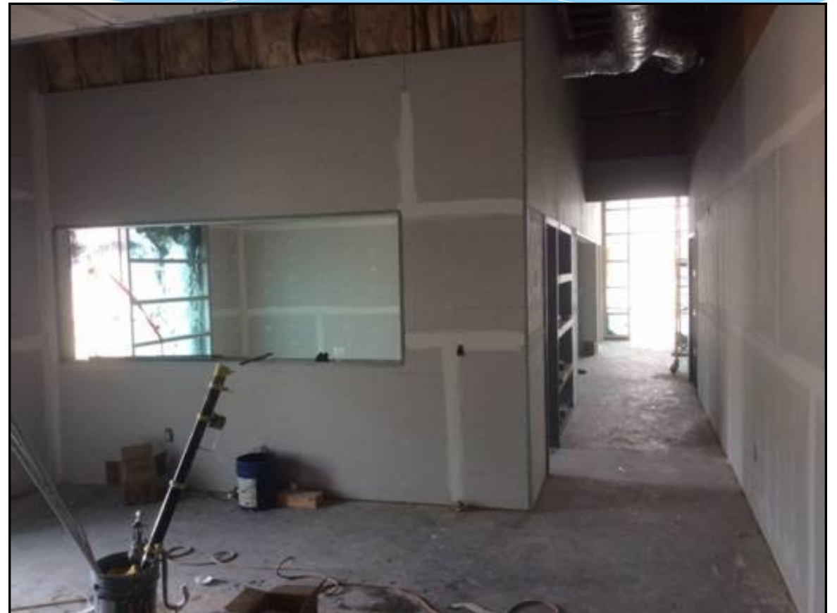
Admin Bldg: East Hallway
