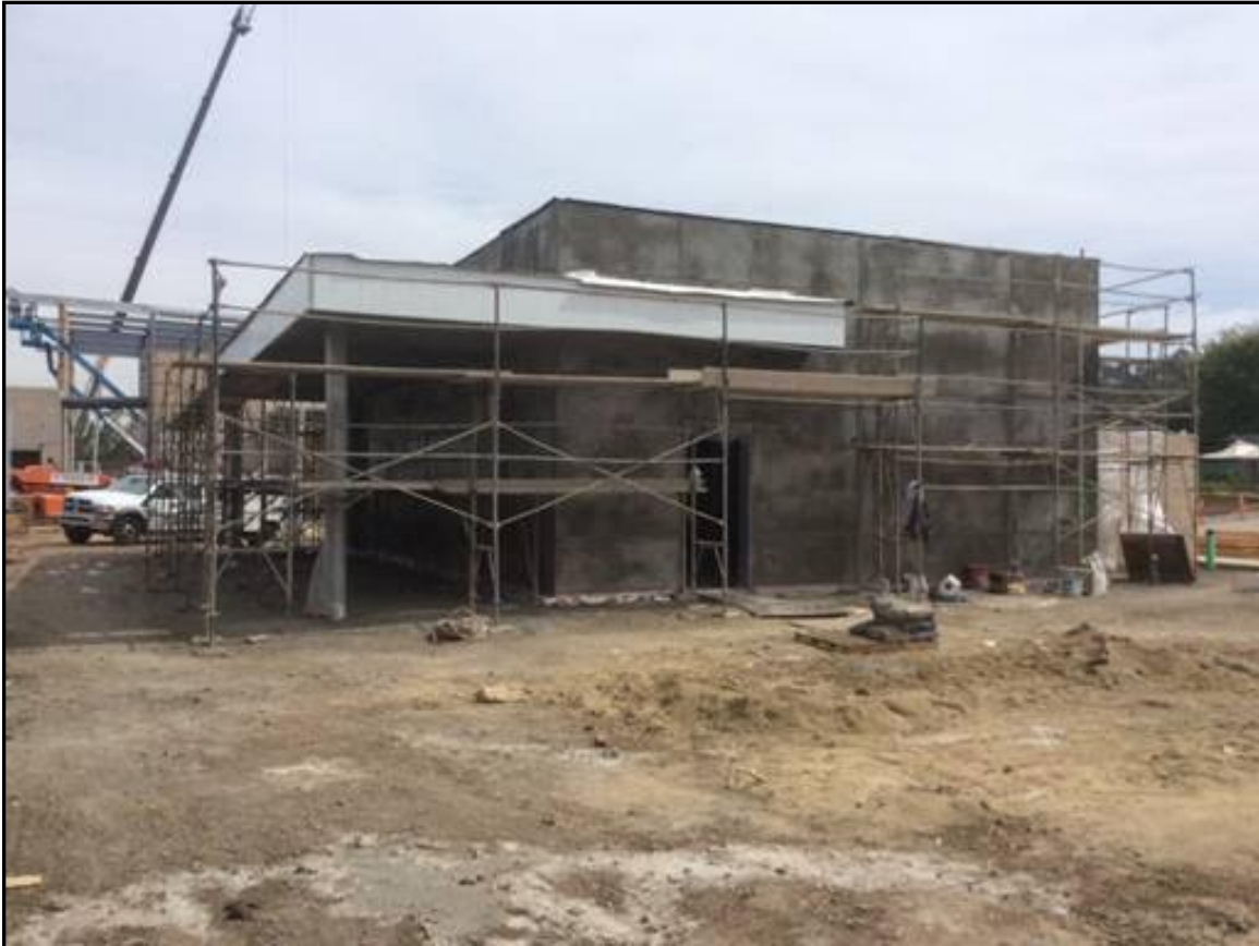
Admin Bldg: West Elevation
