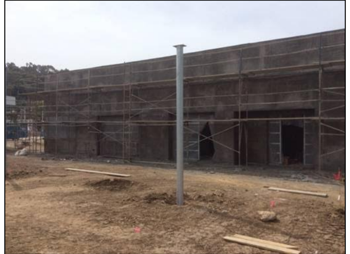
Admin Bldg: East Elevation
